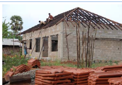
Roof work in progress in the Northern Province. Credit: UN HABITAT
