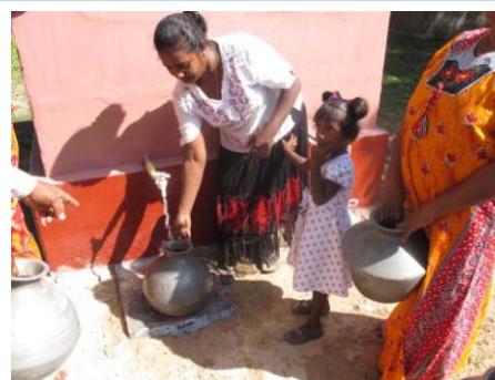
Delft water supply scheme opened for public use on 26 Jan 2012. Credit: UNICEF
